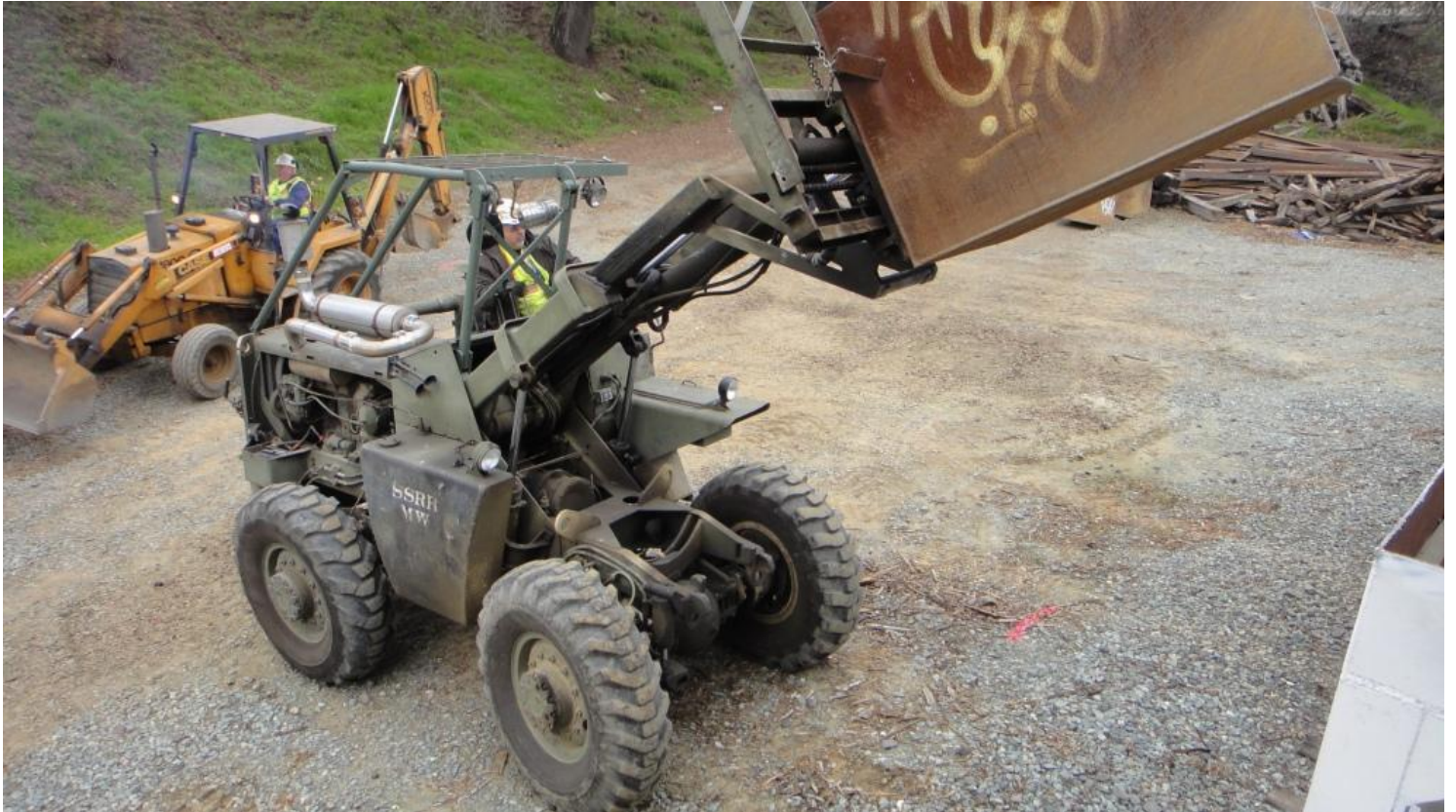
It was a dance of big machines down at Setzer where highly skilled operators Harry on the back-hoe and Mike F. on Big Green fill the hopper cars with rock
