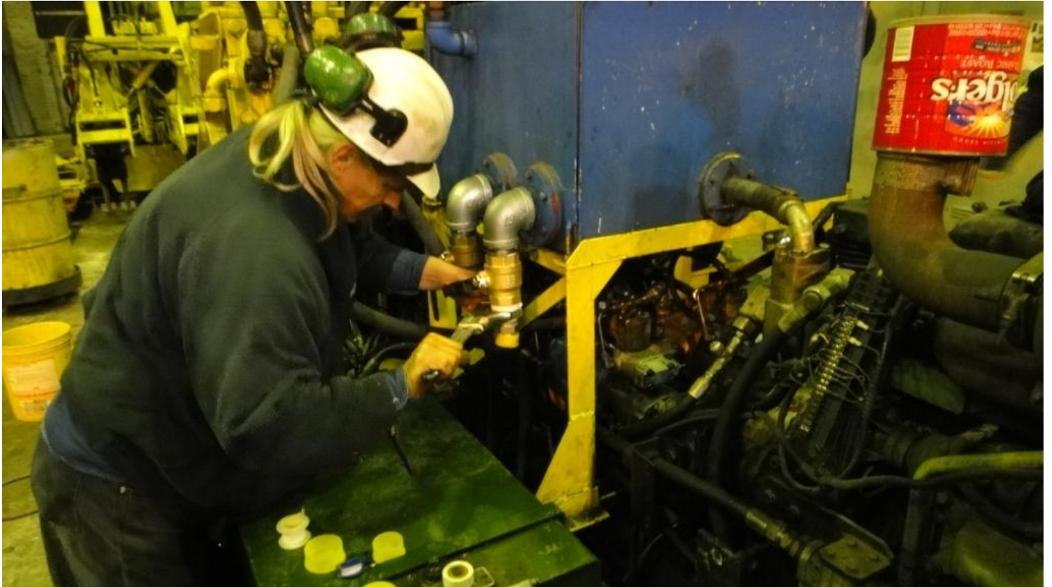
Fred installs a new ball-valve fitting on the hydraulic tank of the tie-shear
