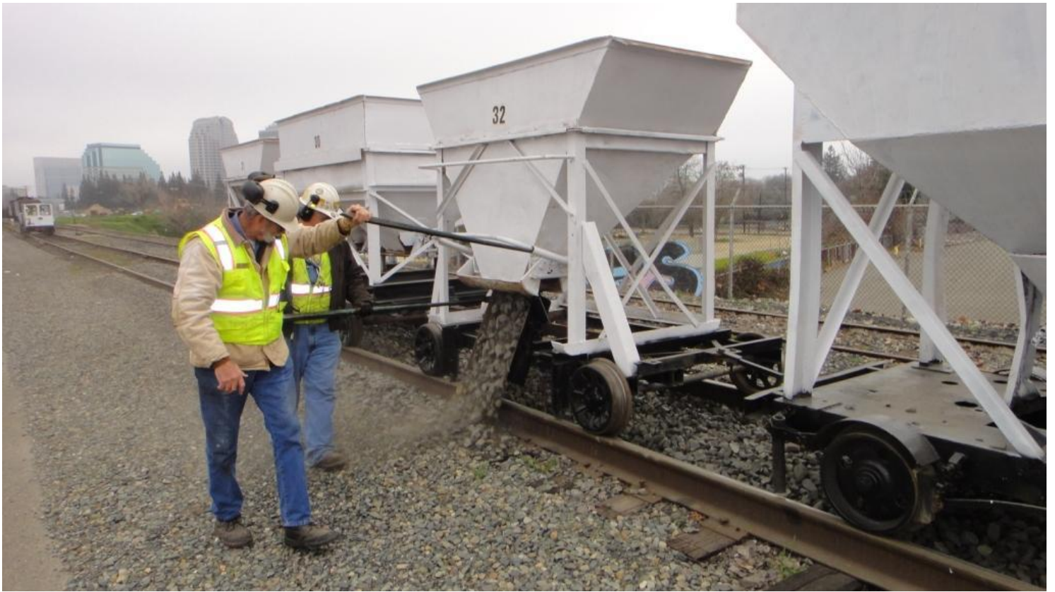
Alan and Mike F. ballasting the west side of the rail
