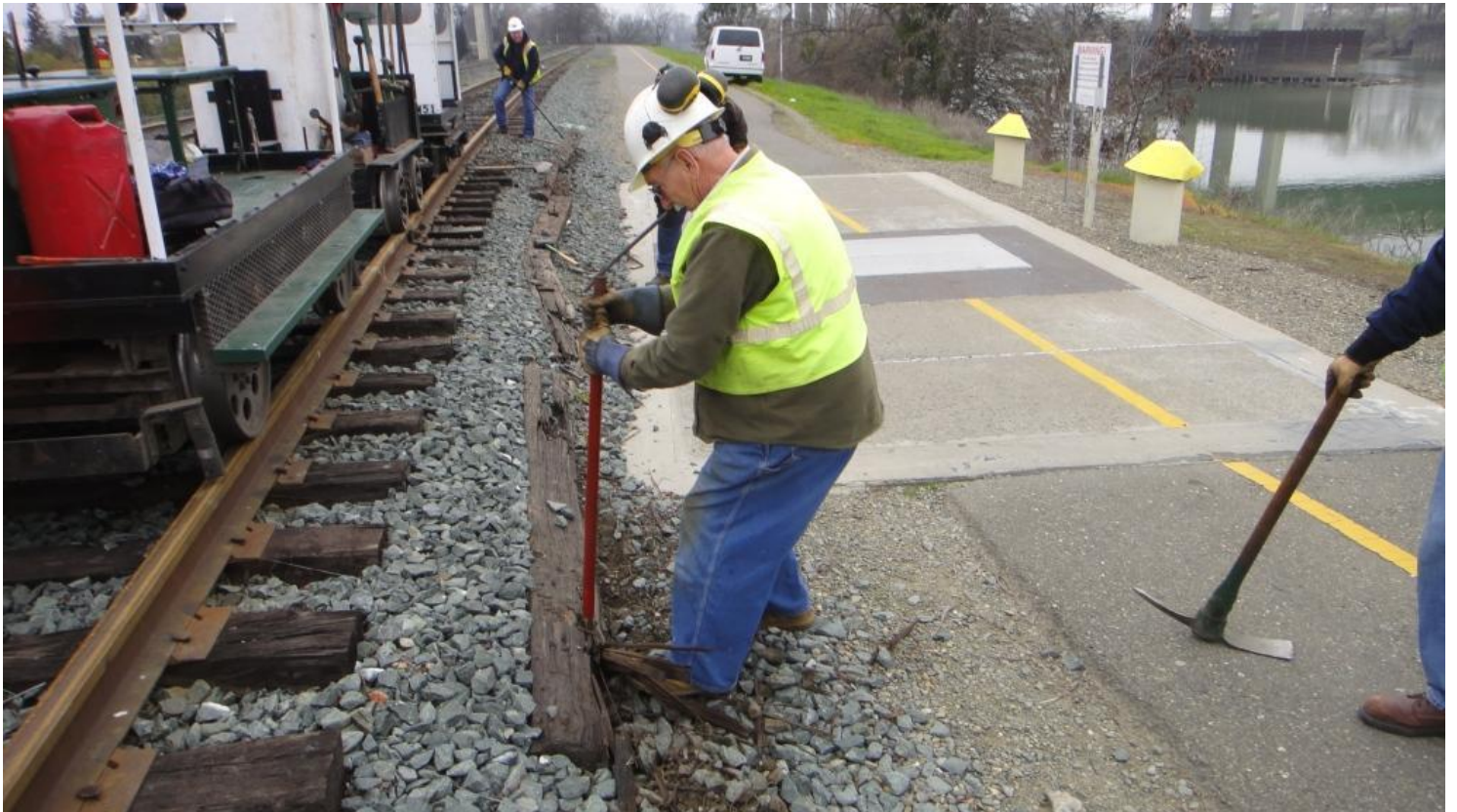
Clem cleverly uses a pipe as leverage to straighten bent rebar
