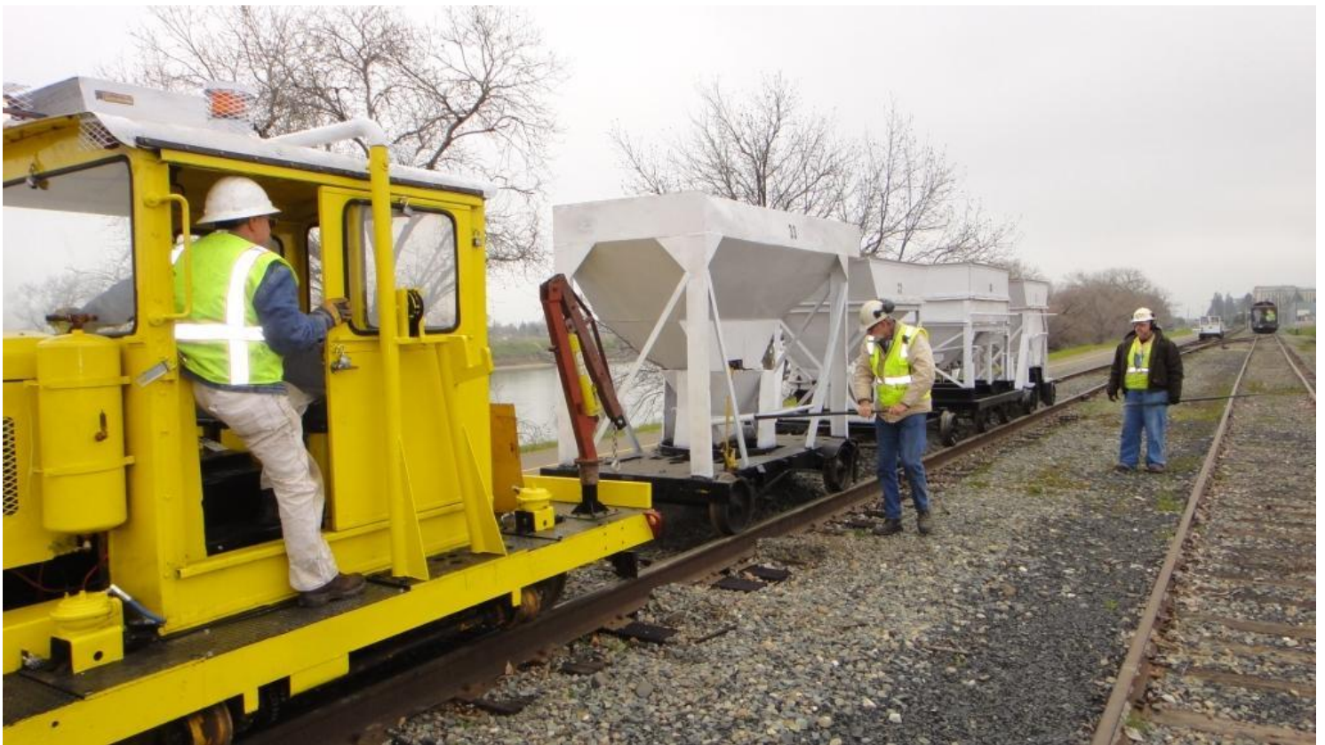
Mike H. pilots the Kalamazoo pulling the four ballast hoppers very slowly as Alan and Mike F. release the rock. The hopper that Alan is unloading is the new one built in our Shops by master welder and metal artist, Cliff Hayes
