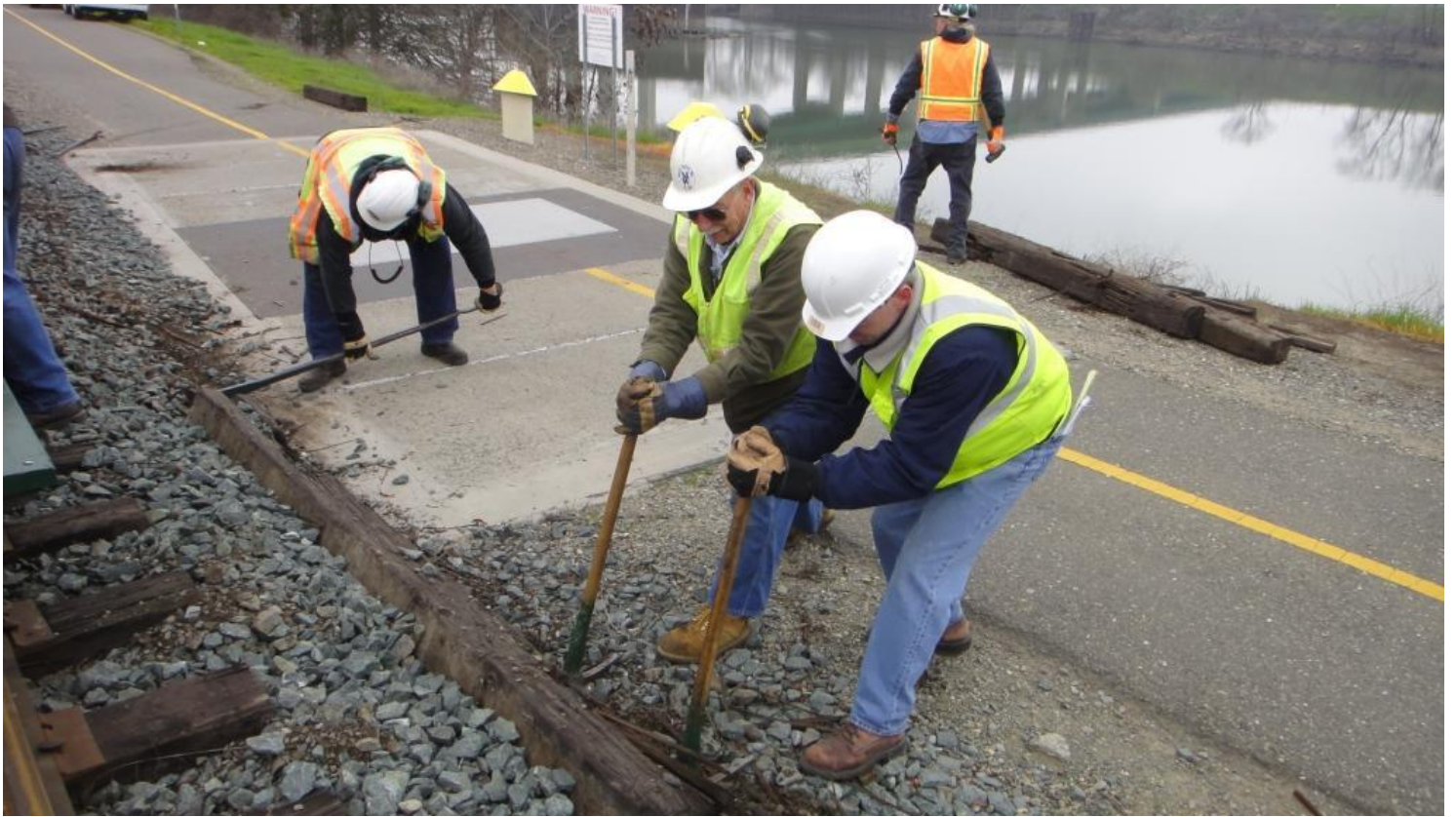
Clem and Kevin use mattocks to pry-up a piece of the old retaining wall
