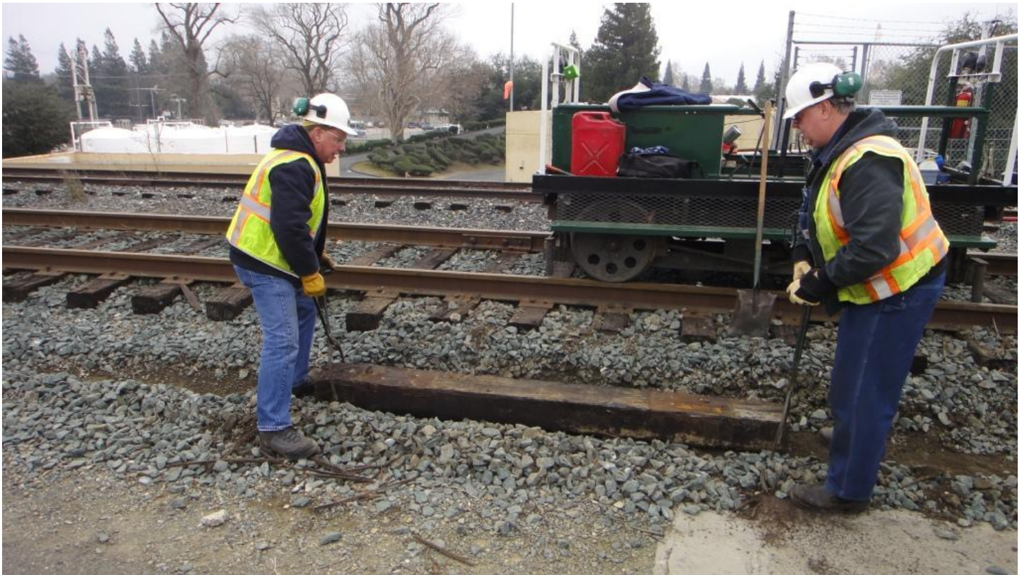
Ed and Chris maneuver a replacement very heavy hardwood tie into place as part of the retaining wall rebuild
